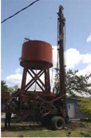
Rig beside water tower
